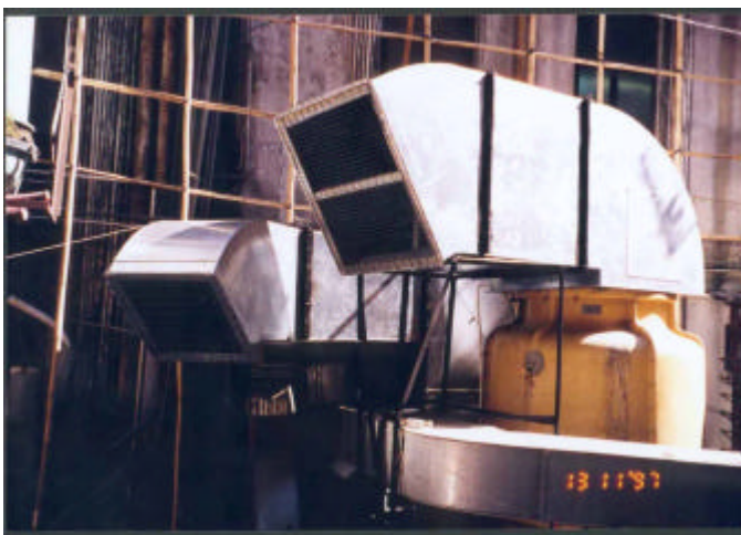
Ventilation system noise reduction works in a Chinese restaurant
