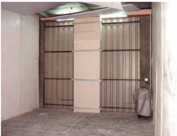
Testing the roof cladding 3060mm X 3300mm
